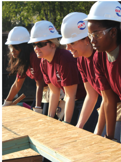
PHOTO COURTESY HABITAT FOR HUMANITY
